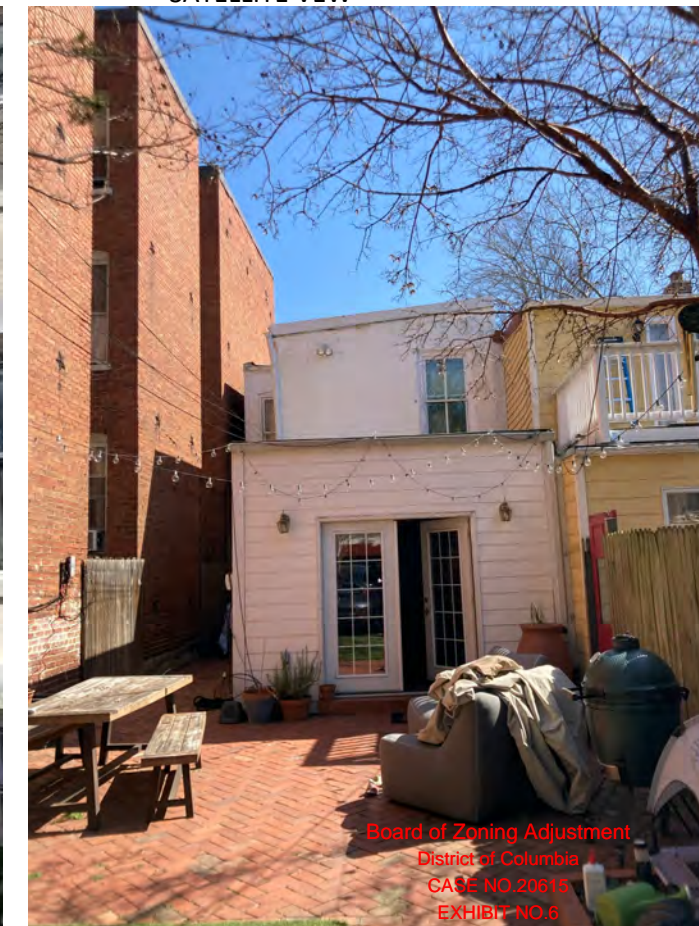
EXISTING REAR FACADE
